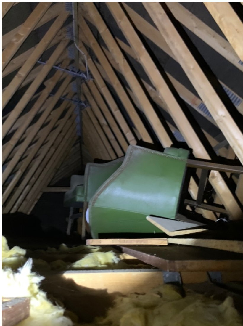
Photo showing roof void
