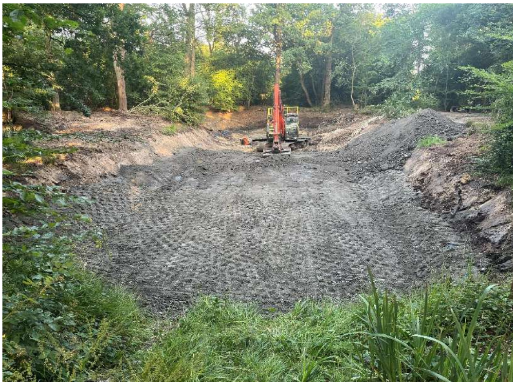
Photograph 5: Clay lining of Lower Pond and compaction in July 2025
