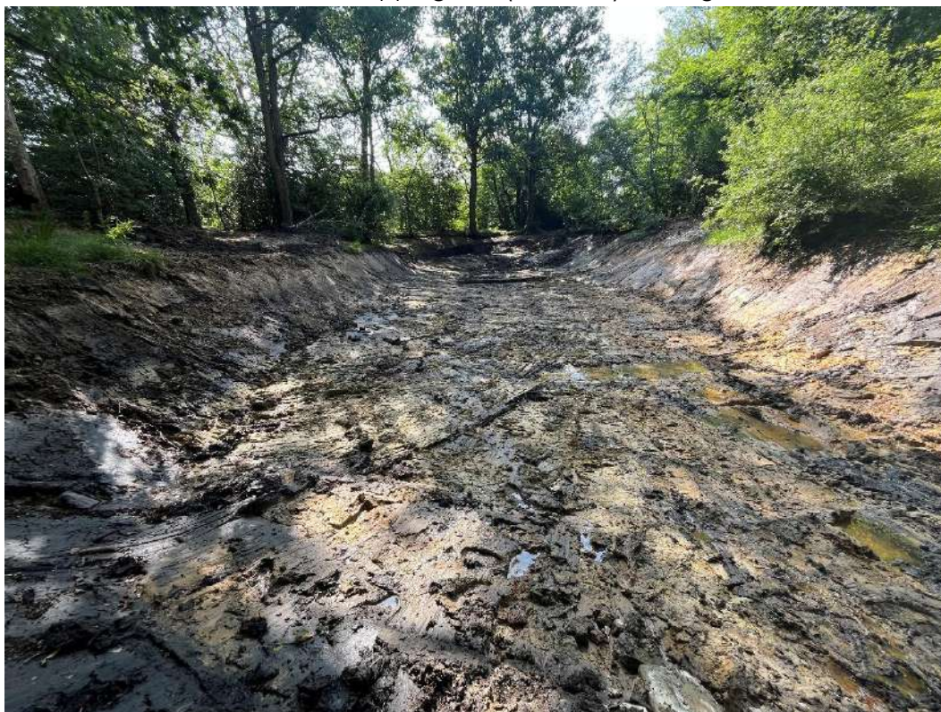
Photograph 4: Lower Greenmoor Pond during silt removal works in July 2025
