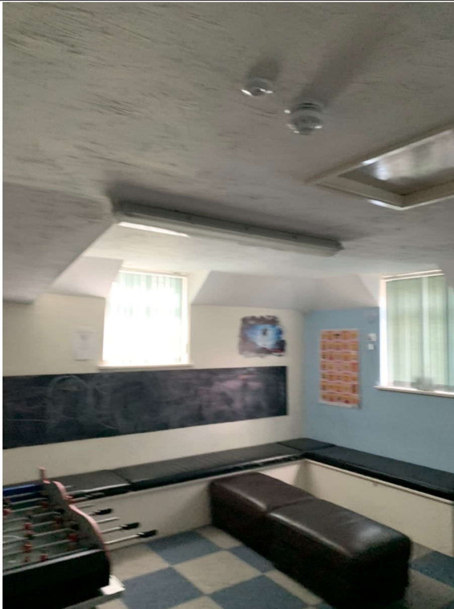
Photo showing textured ceiling coating to the room with inset loft hatch.
