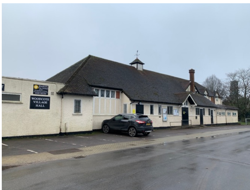
Photo showing front of the property as seen from Reading Road
